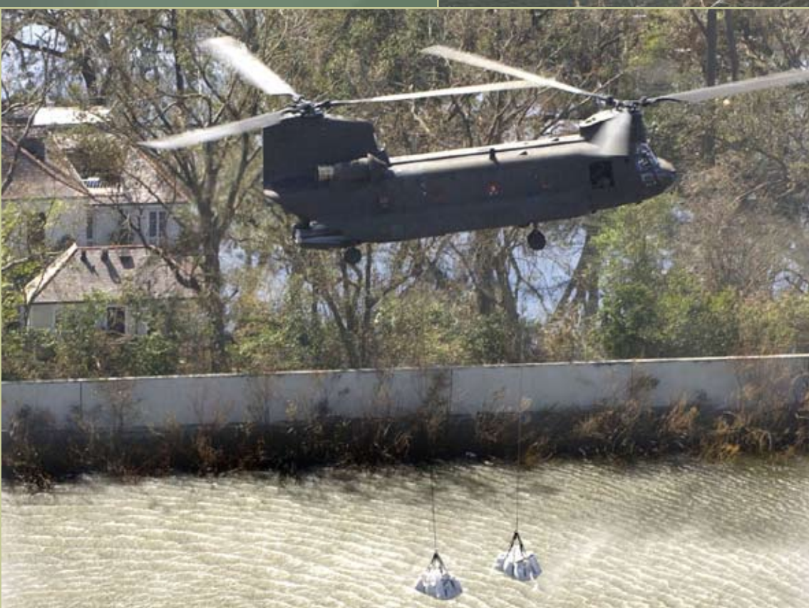
◀ A CH-47 Chinook maneuvers into position earlier this month to drop sandbags into a levee that was demolished when Hurricane Katrina hit New Orleans.
